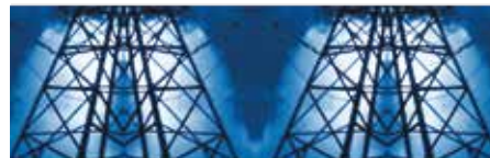
ENERGY SENT ALONG WIRES / Jason Moyes
